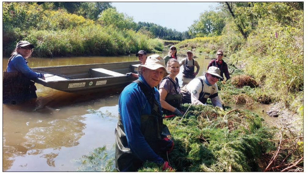
RESTORATION EFFORT – The Nottawasaga Valley Conservation Authority has entered a partnership to restore Willow Creek in the Township of Oro-Medonte. Volunteers installed Christmas trees along the bank of Willow Creek to help with erosion and create habitats for fish.
